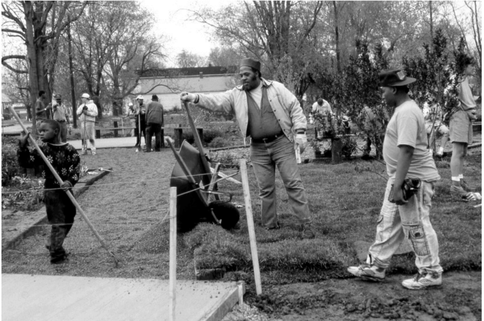
Construction of Illinois Avenue Playground
